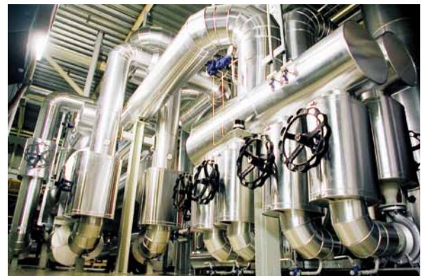
Anlagenverrohrung | Plant pipe-work construction
